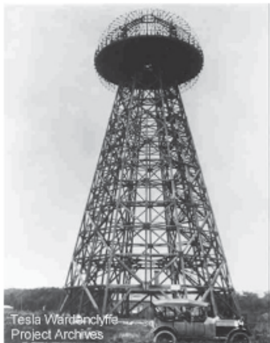
Fig. 18 – The Wardencllyffe Tower (Long Island) in 1903 with steel ribs without copper covering.
